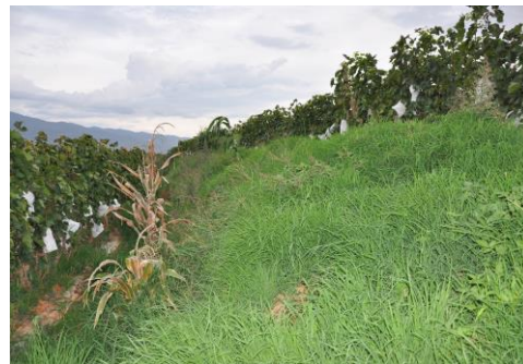
8 (b2) After slope improvement
