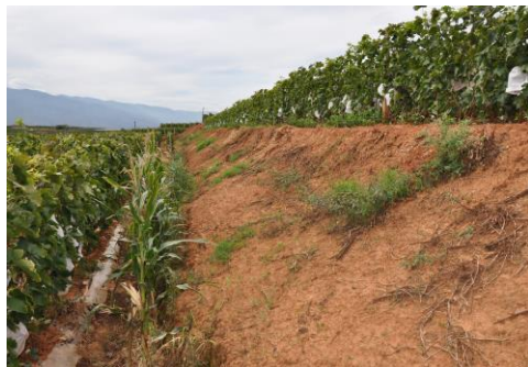
7 (b1) Before slope improvement
